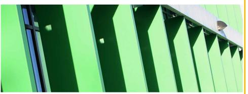
Our aluminium fins are available in a variety of typical profiles and sizes to suit both the structural span and solar shading performance requirements. Finishing options include anodising, polyester powder coated (PPC) finishes to any RAL or BS colour or specialist coatings to mimic natural materials such as timber or terracotta.
