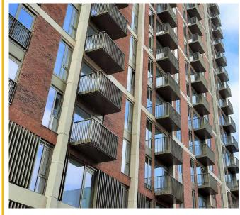
Levolux Sereniti balconies are manufactured in the UK and delivered as pre-assembled units. They will arrive complete with all connections, structural frames, decking, glass or aluminium balustrades, fascias, soffits and drainage solutions.
