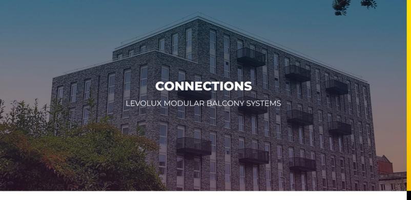
A key performance requirement of any balcony system is the rigidity of the pedestrian surface. Levolux's balcony specifications are designed to ensure that the cast-in connection, first fix bracket, structural frame and pedestrian surface deck combine to limit any deflection to 5 mm or less.
