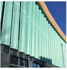
A range of fixed or controllable solar shading fins. A variety of shapes are available, including aerofoil, box and circular. Material choices include aluminium, glass and timber. Secretfix options are available.
