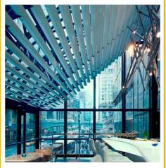
A range encompasses fixed brise soleil systems and a roof shading rack arm system that can be controlled manually or mechanically in conjunction with a control system.
