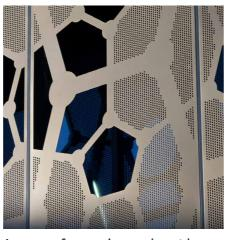
A range of screening and vent louvre systems as well as architectural perforated panel systems that can be used to screen car parks and other structures for aesthetic and/or solar control purposes.
